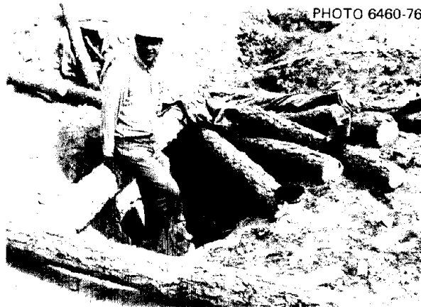
Fig. 5.5. Wrecked entry of Russian Pole-Covered Trench Shelter at 20 psi.
